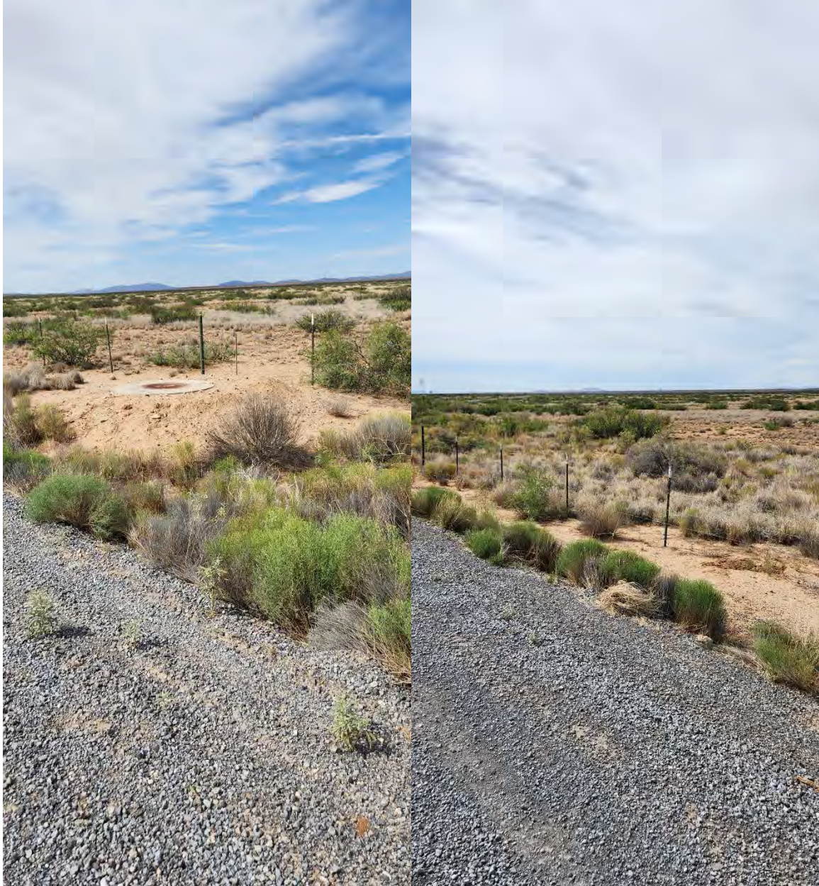
Figure 7. View of maintenance hole cover and landscape along access road between proposed parking lots.
