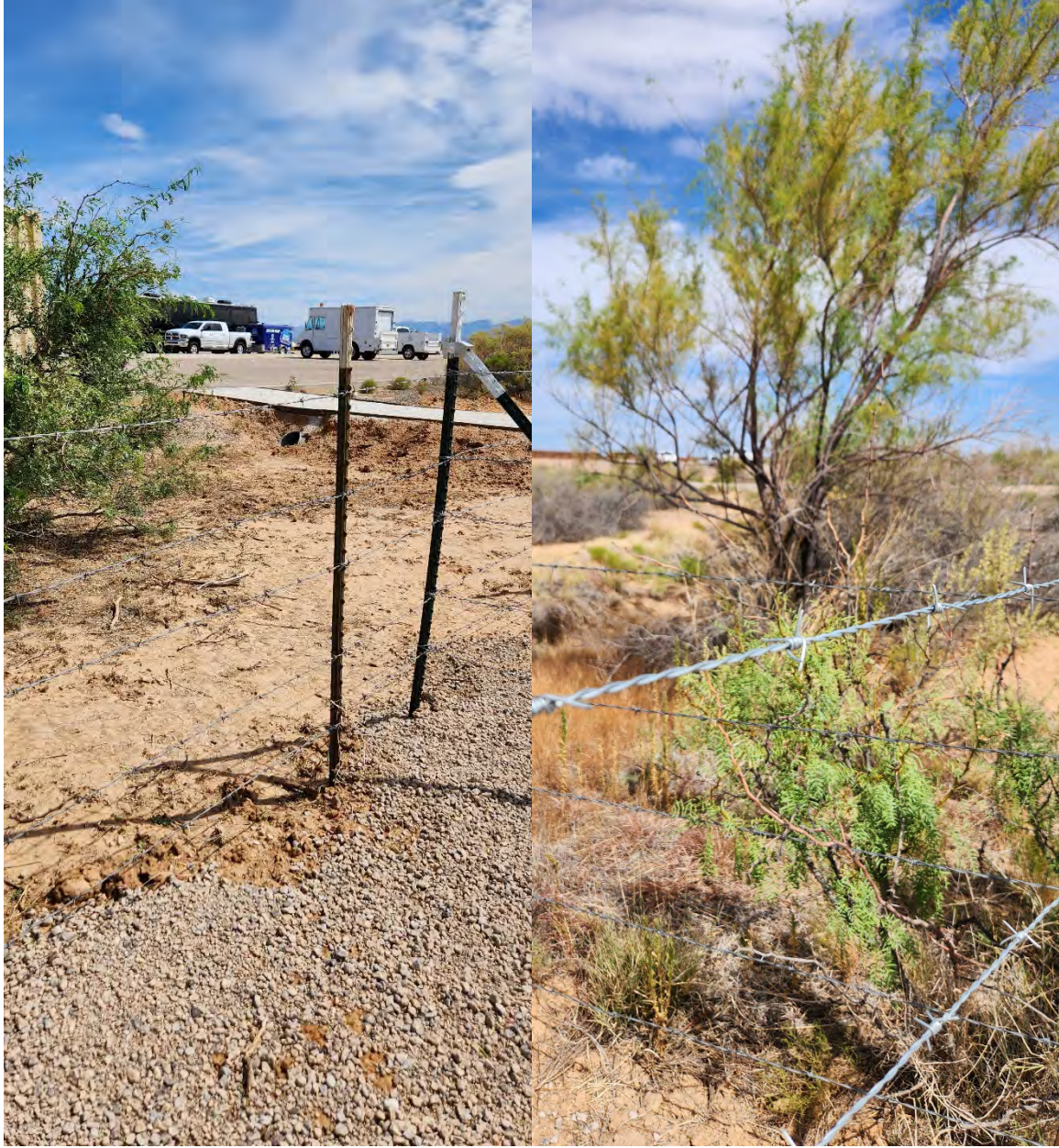
Figure 1. View of small culvert southwest of existing parking lot and vegetated area next to culvert.
